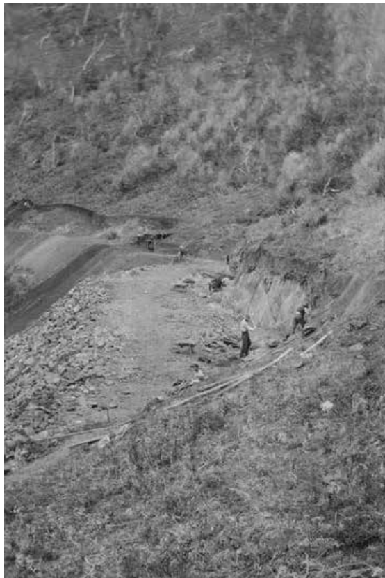
'Diggers constructing Ocean Road'. The Great Ocean Road was built as a tribute to soldiers of the First World War. Surveying of the road commenced in August 1918 and construction in 1919. Thousands of veterans were employed for the construction, using picks, shovels and horse-drawn carts. The road was officially opened on 26 November 1932.
