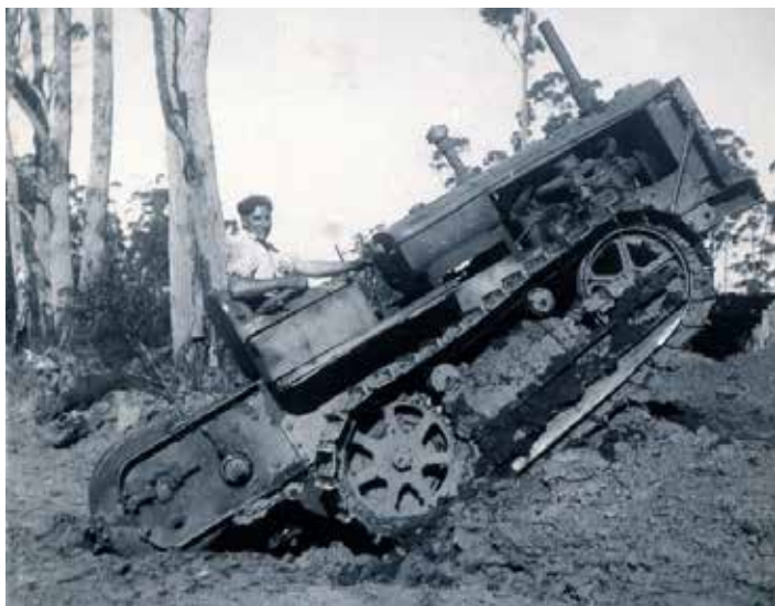
Erwin Snr On Babington's First Bulldozer
