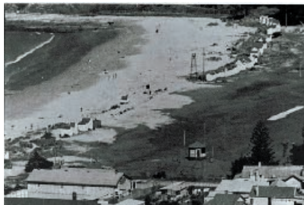
Another view of the original complex showing its proximity to the beach. Notice the band stand and bell tower c.1937.
