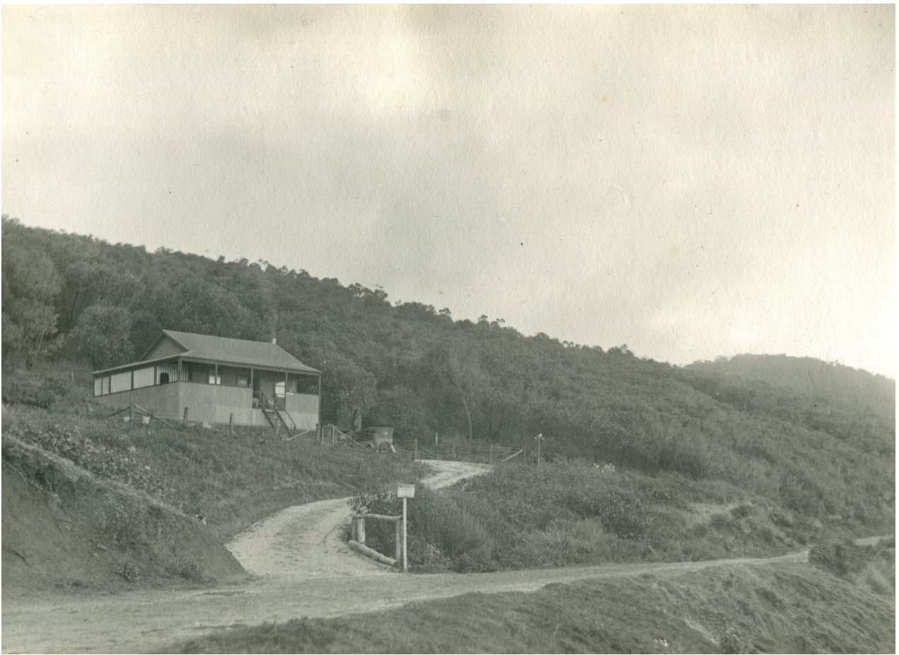
Summerhill the cottage 1930s – extension to the left-hand side (image: Early North Iorne002 – Alan Doyle)
