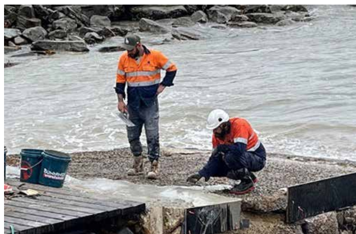
Contractors patching up the ramp
